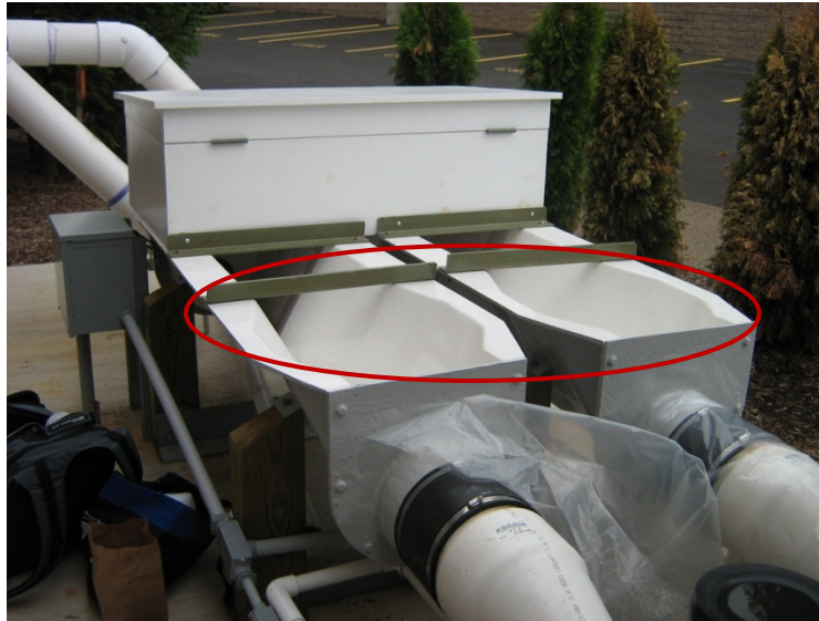
Figure 3-8 Two flumes (circled) for discharging stormwater runoff (Giant Eagle)
