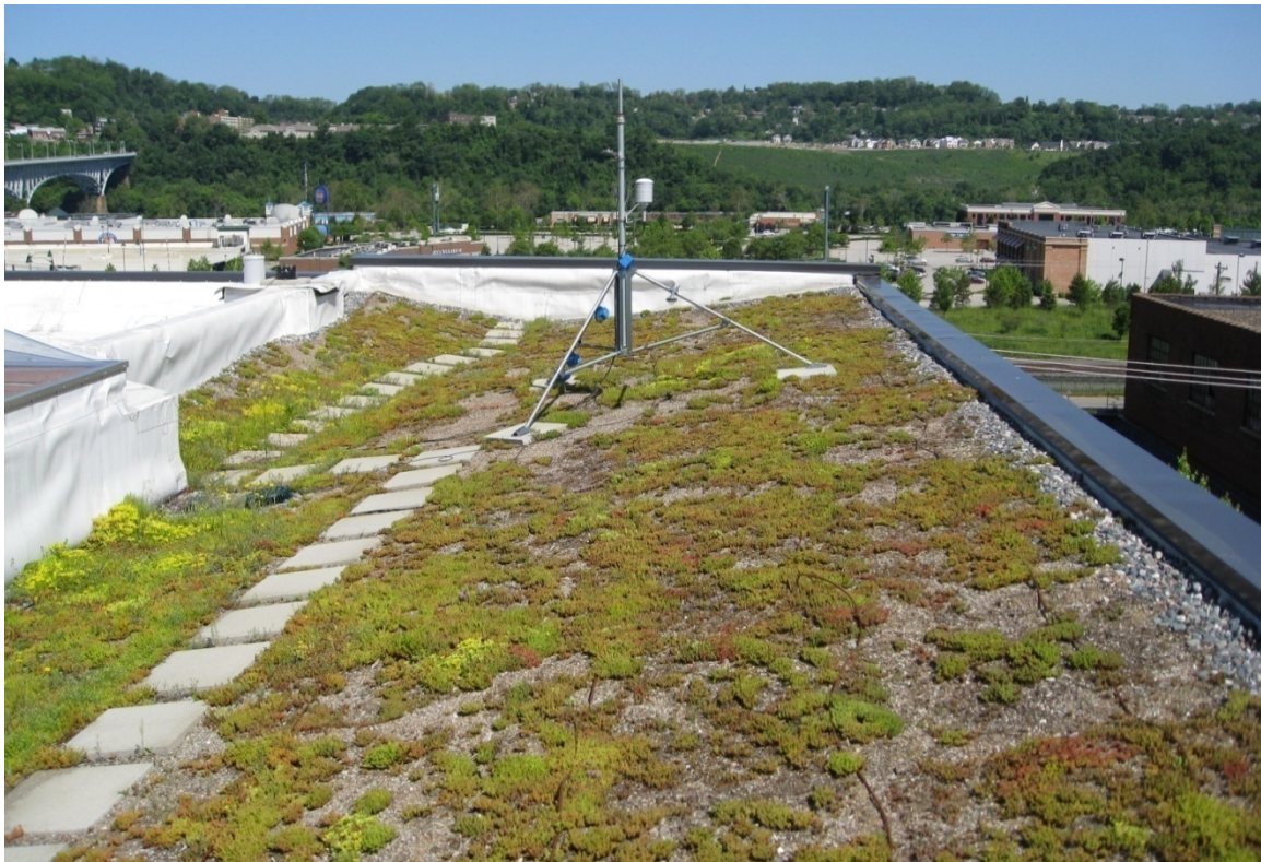
Figure 3-16 GLT Green Roof at Homestead
