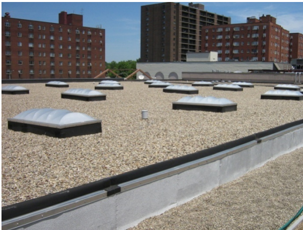
(a) Control Roof
