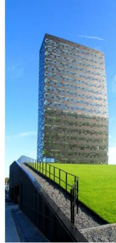
(c) FiftyTwoDegrees Business Innovation Center (Nijmegen, The Netherlands)
