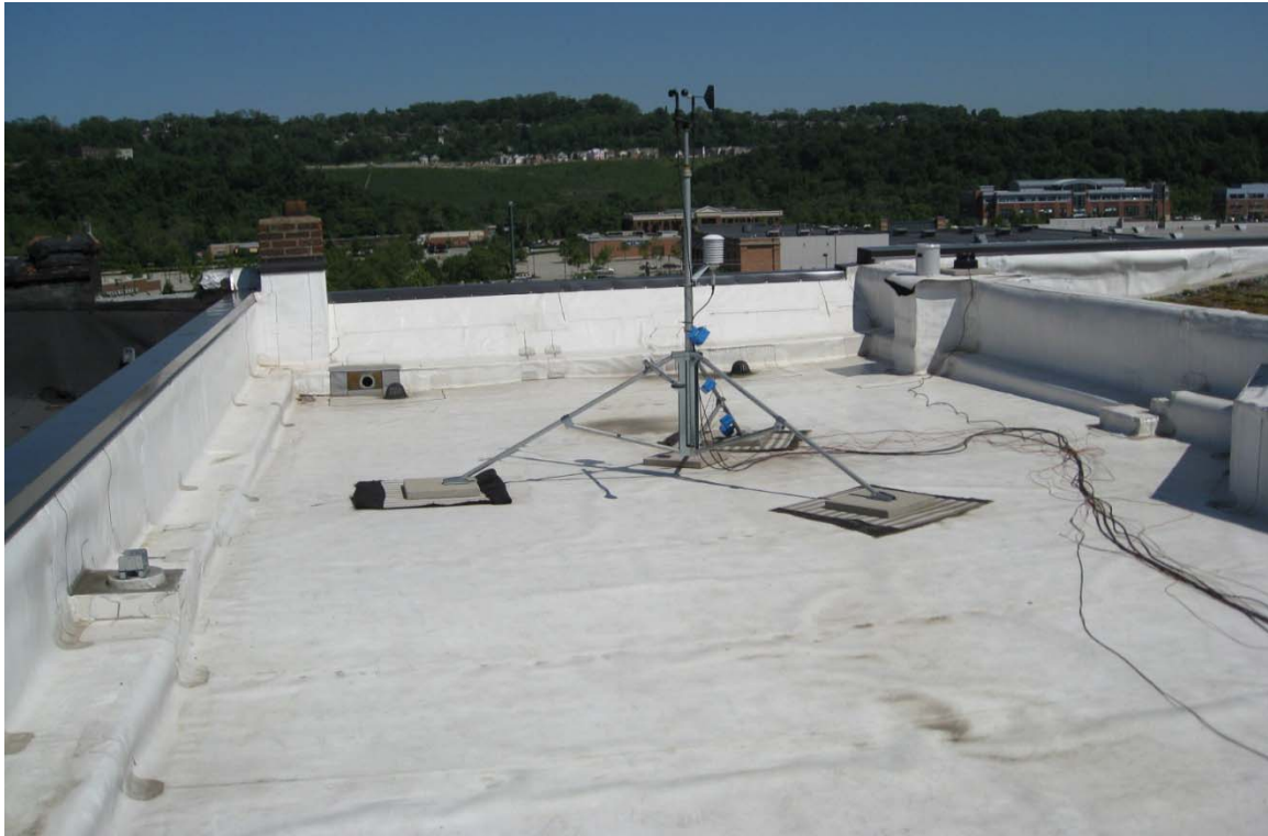
Figure 3-17 Control Roof at Homestead
