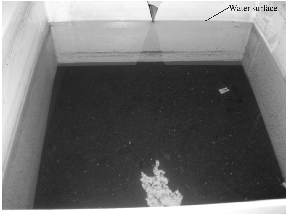
Figure 6-22 Runoff water from control roof stored in the weir box (Homestead)
