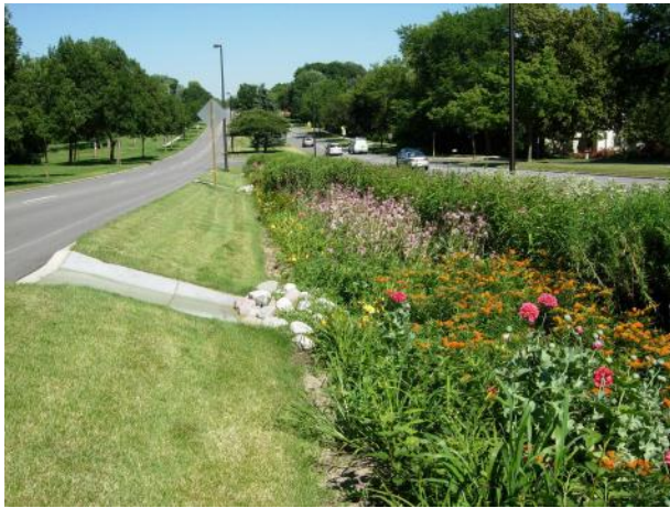
Figure 4-1. Bioretention in Median
