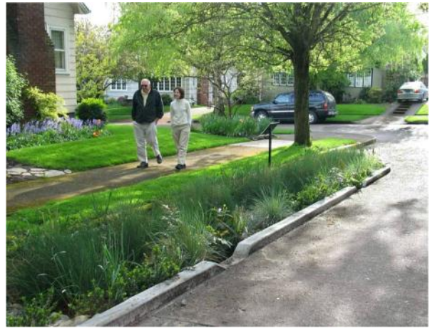
Figure 4-2. Curb-extension Bioretention
