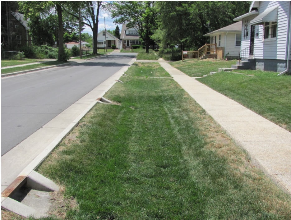
Figure 6-1. Bioretention Planted with Turf Grass
