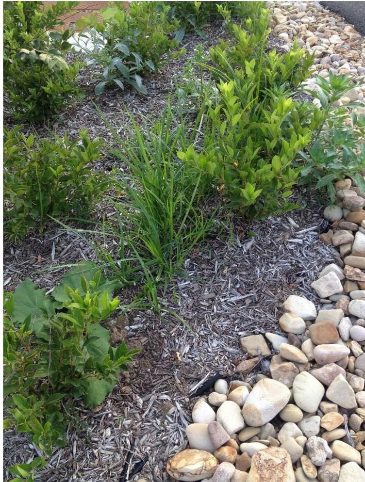
Rain garden short circuit and excessive siltation from parking lot runoff. Not enough water is going to enter this rain garden to do any good. Notice the fouling of the surface.
