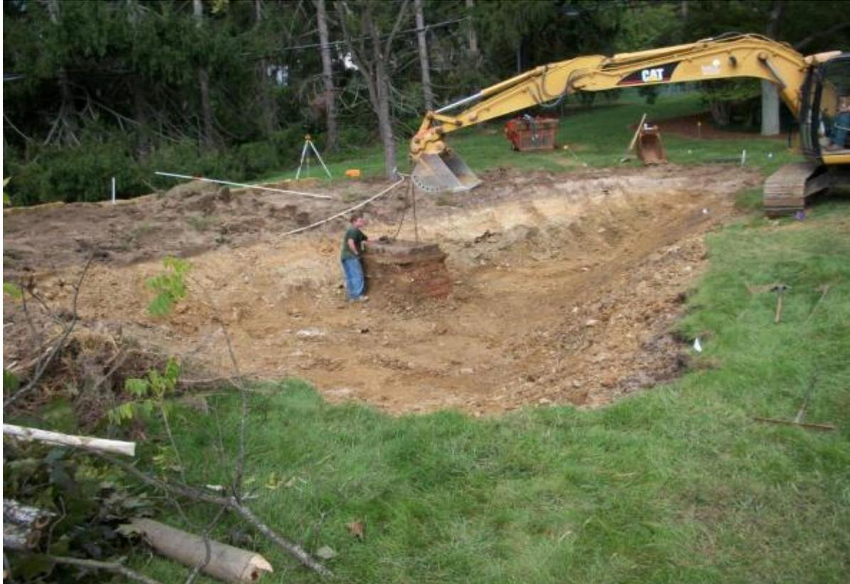
The contractor should be able to reach into the area without entering it which avoids compaction.
