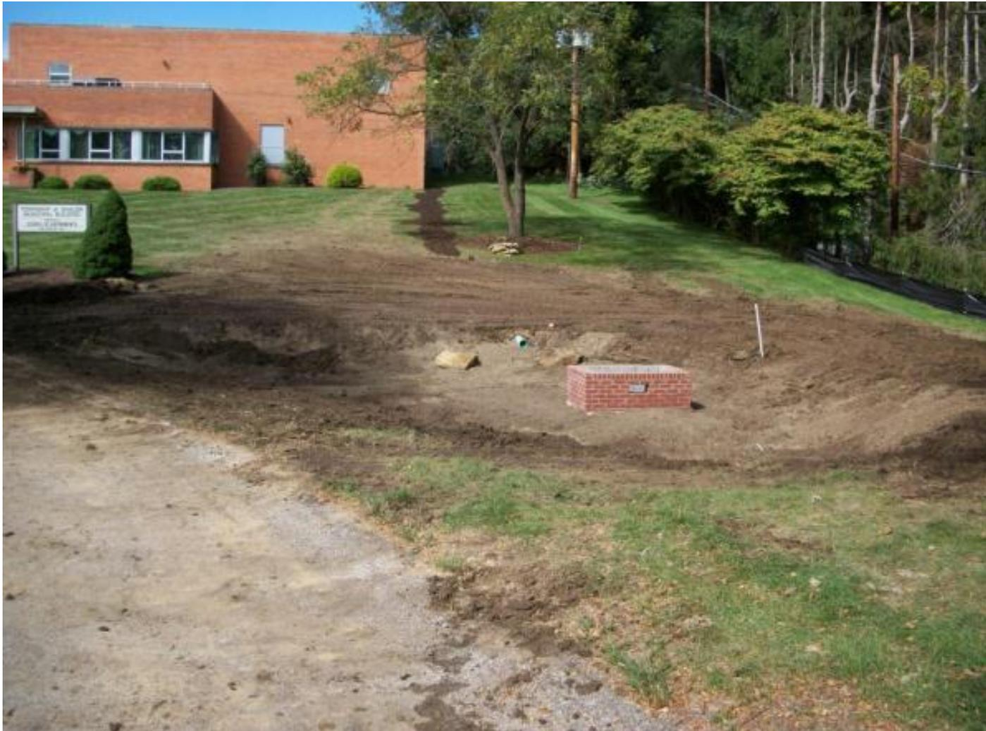
Planting needs to be done quickly after the infiltration soils are placed. Do not allow the soils to sit for months getting fouled with silt.
