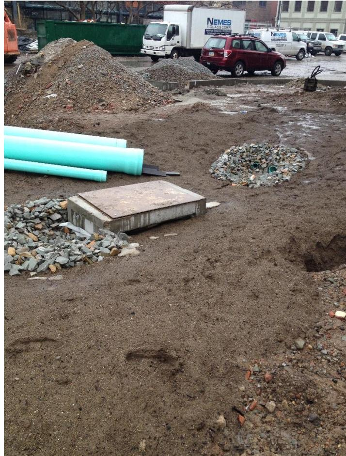
This is a problem with project sequencing. The only good solution is to remove the geotextile and replace if you are forced to use the stuff.
