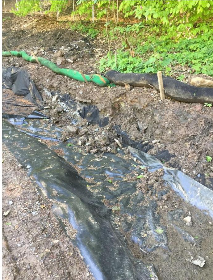
Here is a well protected trench pre-soil. We were able to get the design team to switch the geotextile to straw.
