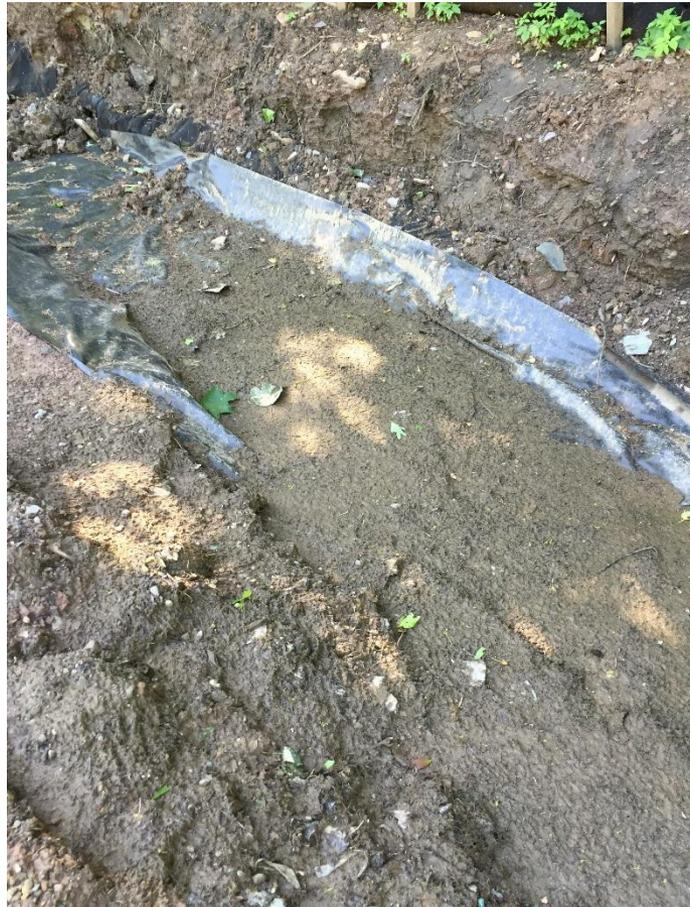
Plugged geotextiles are the enemy of good infiltration.
