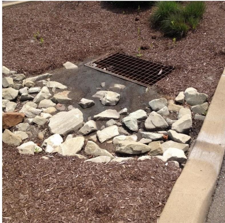
Erosion is a common problem, these curb cuts are too small. The solution would be to make them larger and farther away from the inlet.
