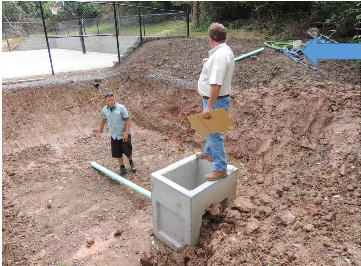
Ground water in the bottom of the excavation is a bad sign.
