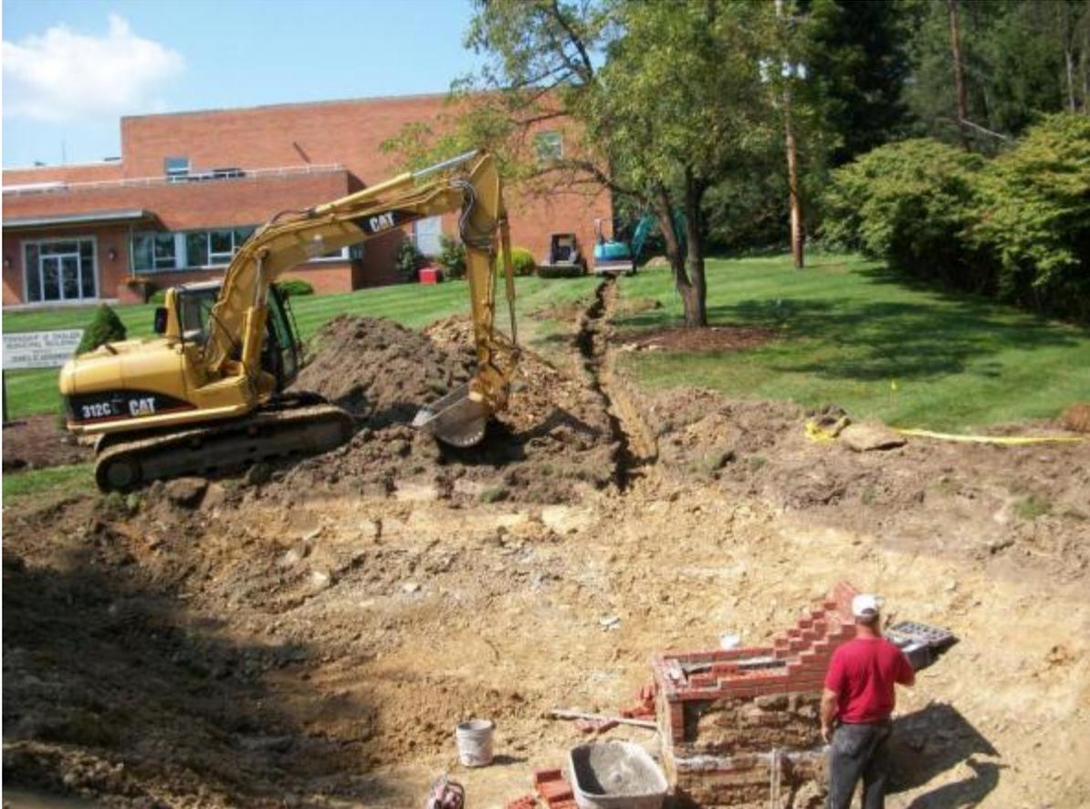
Notice the excavated area is not being occupied by heavy machinery.
