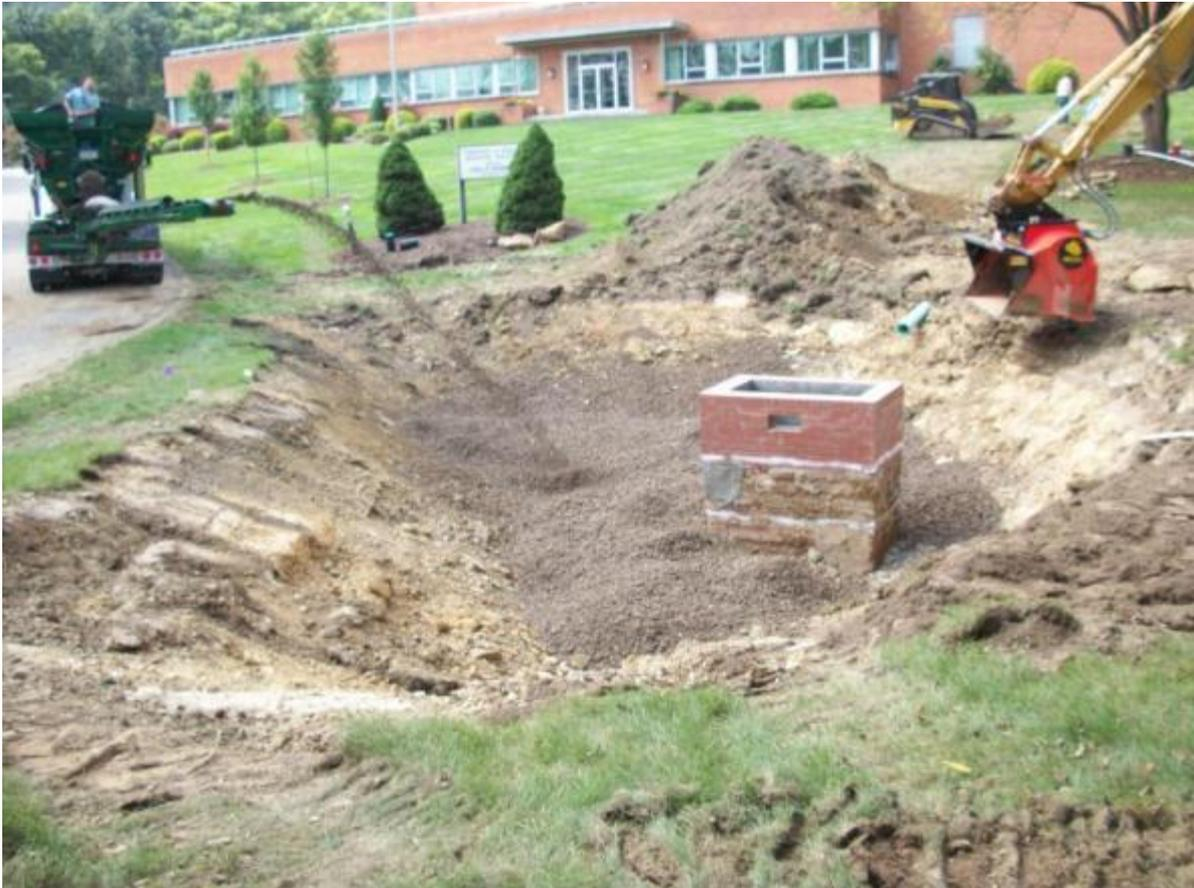
Again, no equipment is in the RGA causing compaction.
