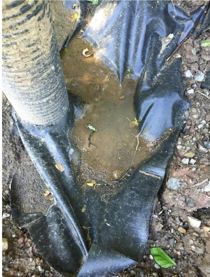
This geotextile was fouled despite silt sock barrier.
