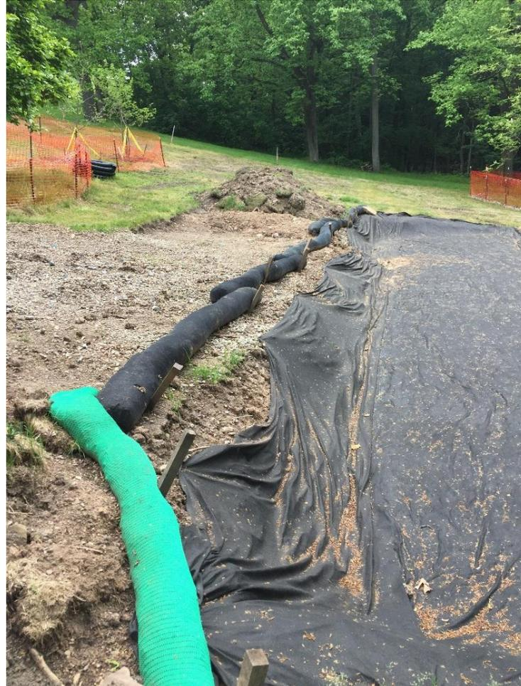
This is an exfiltration trench, water is coming from the street into this gravel “tank” and then infiltrating into the soils. We were not worried about the fabric plugging here.
