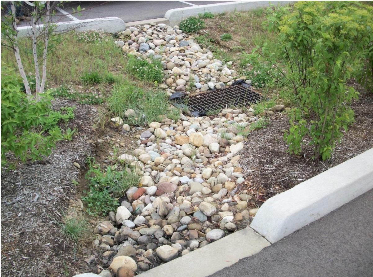
Armoring the edge prevents erosion but be careful not to dam out the sheet flow.
